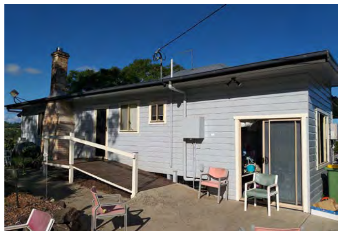
Figure 56: View of the rear addition. Source: TZG Heritage, 2024.
