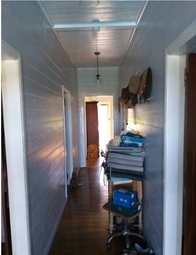
Figure 61: Main corridor showing early internal finishes retained. Source: TZG Heritage, 2024.
