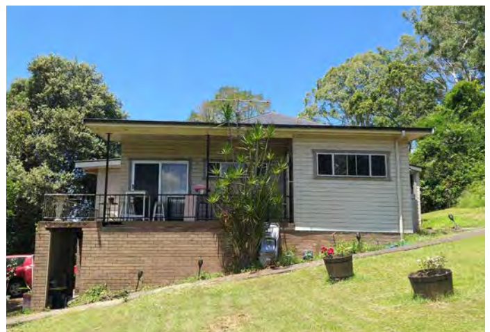
Figure 70: View of the house facing south. Source: TZG Heritage, 2024.
