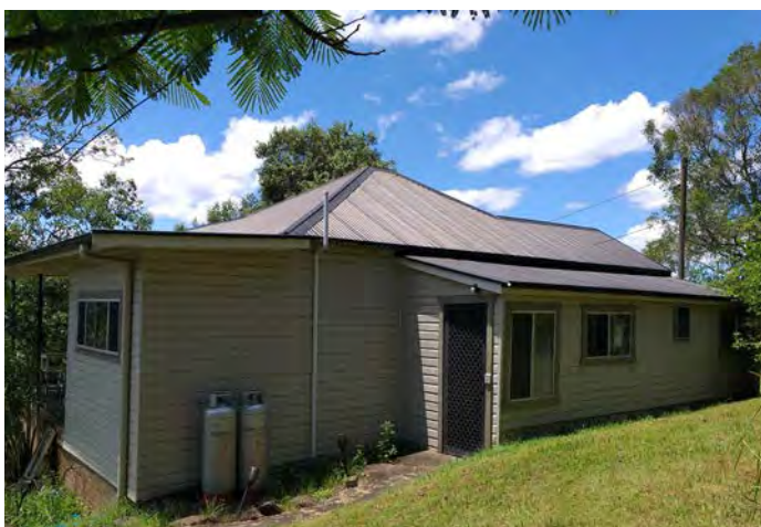
Figure 71: View facing east. Source: TZG Heritage, 2024.
