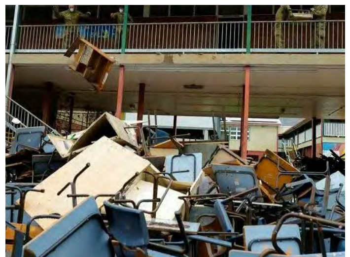
Figure 10: Damage caused in the aftermath of the 2022 February flood.
