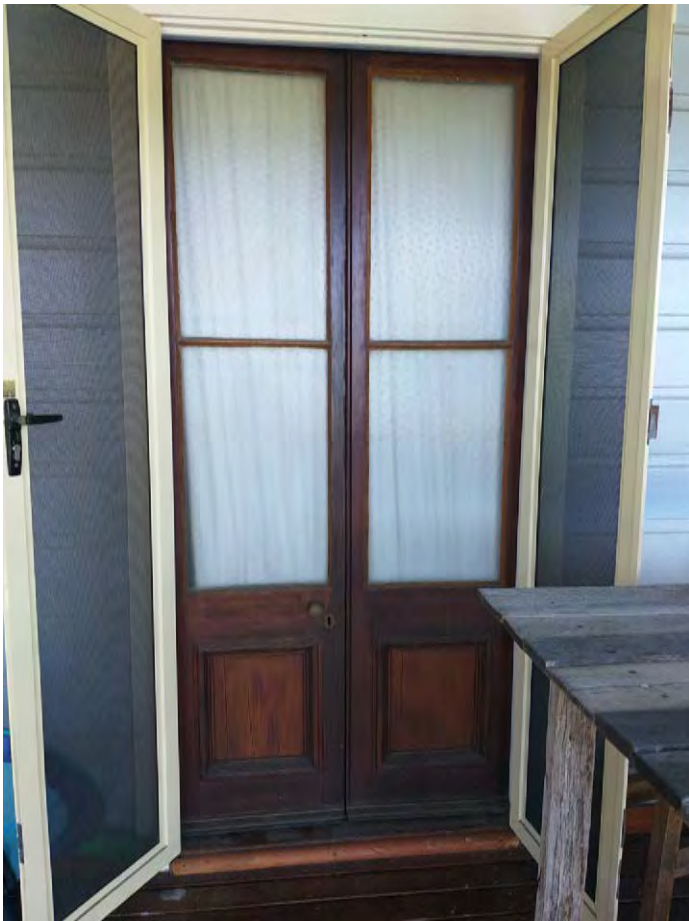
Figure 59: French timber doors behind aluminium framed screens. The doors are believed to have been constructed from local cedar. Source: TZG Heritage, 2024.
