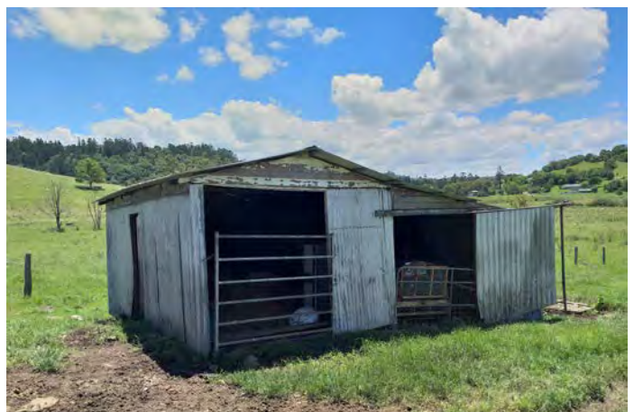
Figure 75: Storage Shed. Source: TZG Heritage, 2024.
