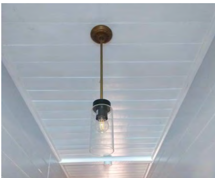
Figure 63: Detail view of timber board lined ceiling. Source: TZG Heritage, 2024.
