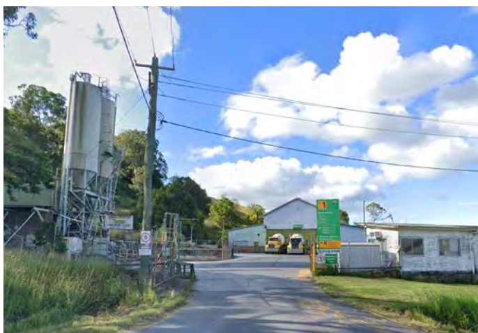
Figure 50: North Lismore Boral Concrete plant at the corner of Lake Street. Source: Google Streetview.
