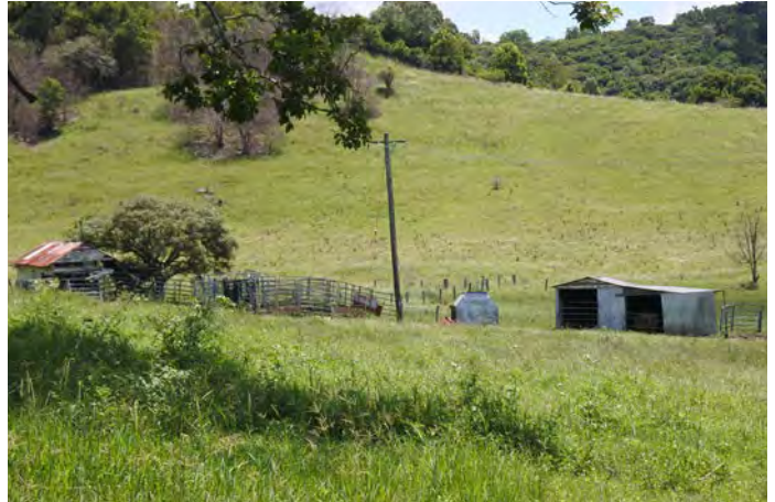
Figure 73: View of remnant farm outbuildings. Source: TZG Heritage, 2024.
