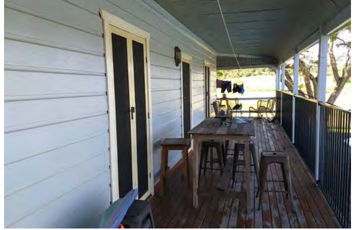
Figure 58: View facing north from the reconstructed verandah. Source: TZG Heritage, 2024.
