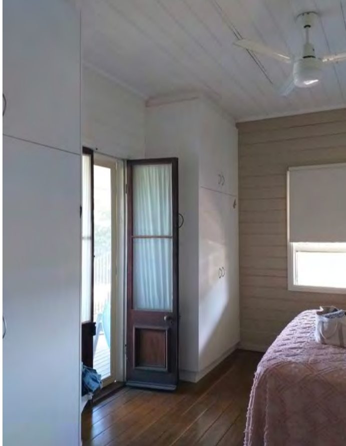
Figure 65: Original timber board lining and floorboards in the main bedroom. Source: TZG Architects, 2024.
