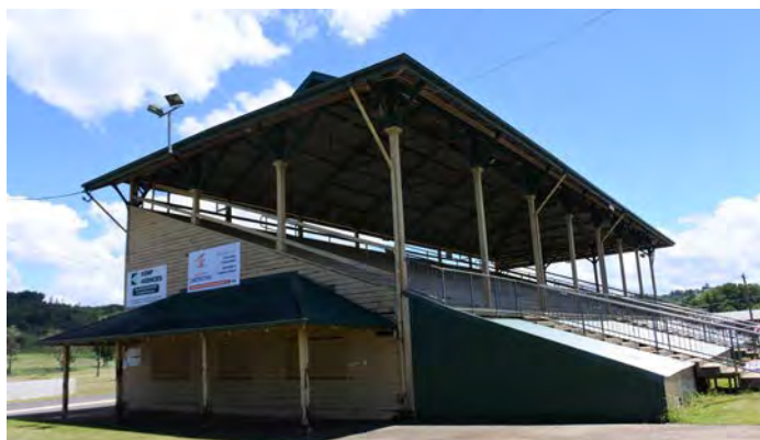
Figure 51: Grandstand building at Lismore Showground. Source: TZG Heritage, 2024.
